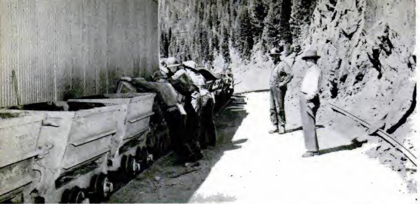
Men unload ore cars by hand because demand for cobalt was too great to wait for automatic dumping outfit
